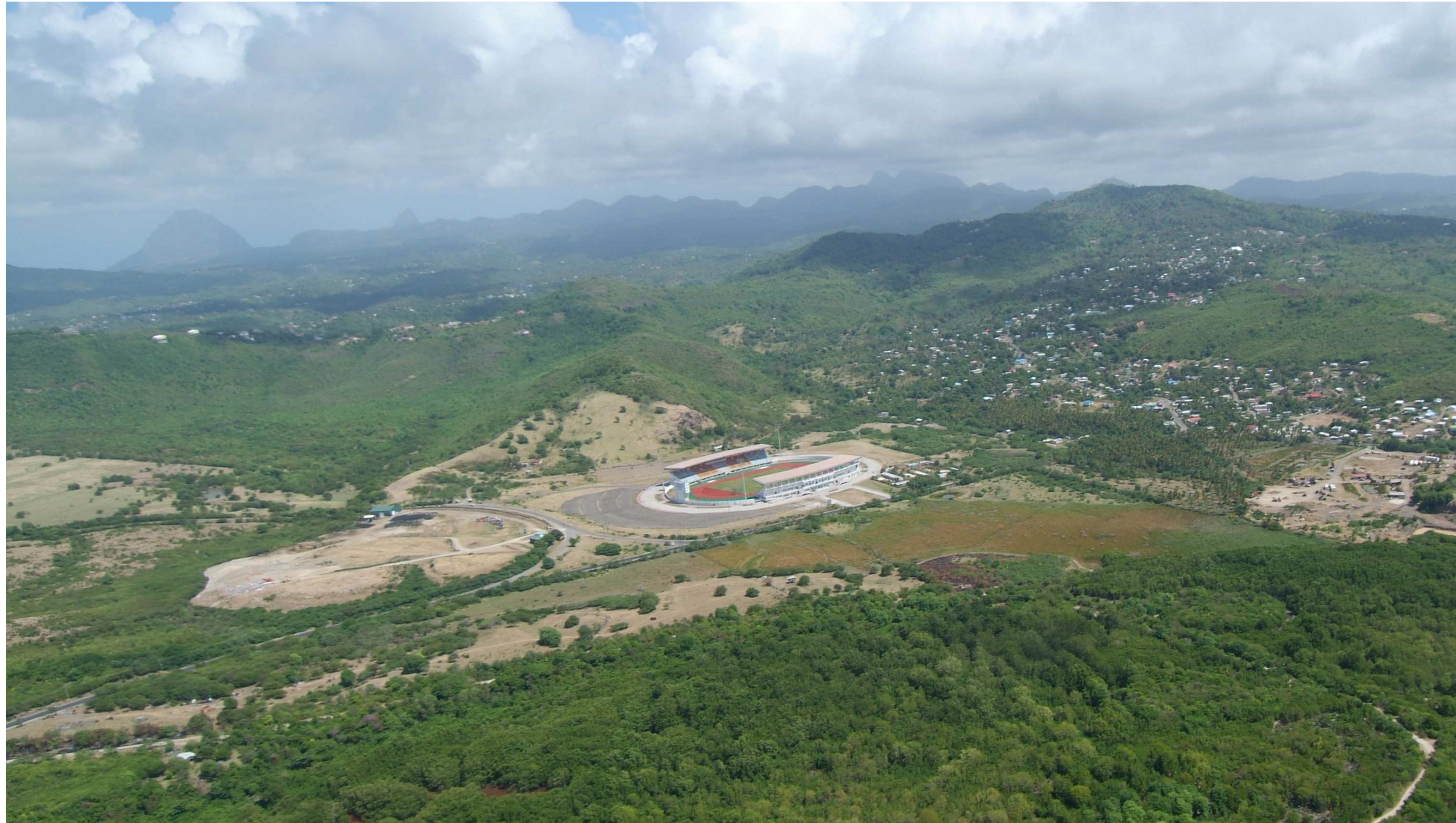
VIEUX FORT NATIONAL STADIUM PHOTO
