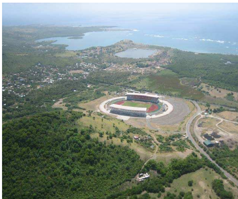
VIEUX FORT NATIONAL STADIUM
