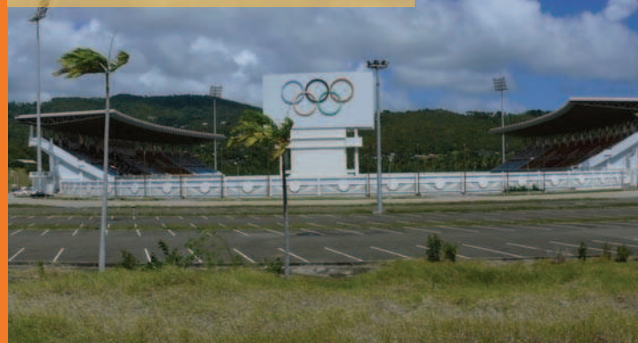
VIEUX FORT NATIONAL STADIUM
