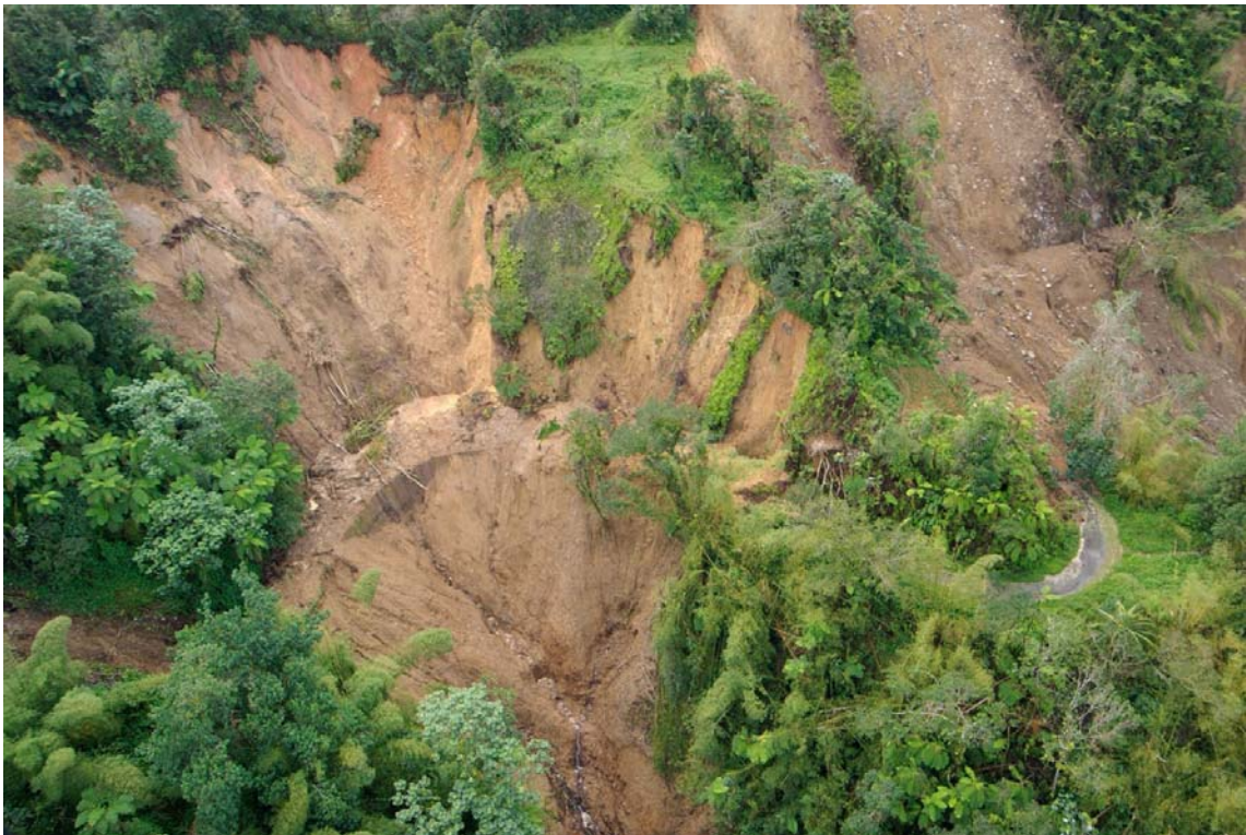
Agricultural access road Migny to microwave tower-II
