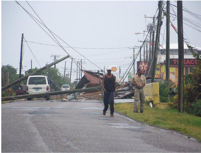
Photo 2: Damaged electrical infrastructure
