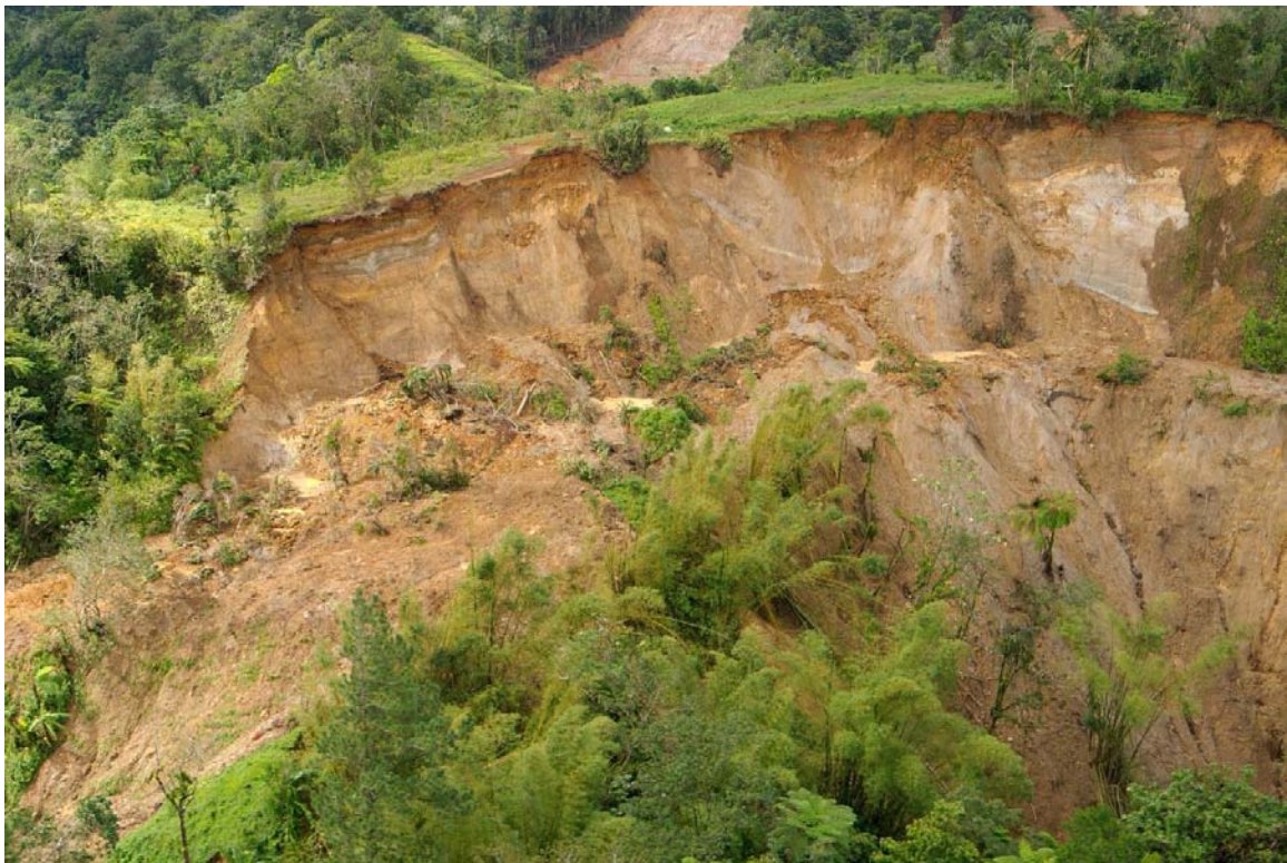
Agricultural access road Migny to microwave tower-I
