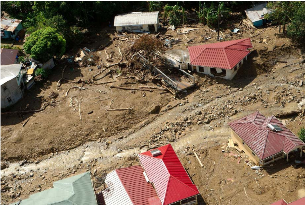
Fond St Jacques: Flow slide burying roadway and dislodging bridge
