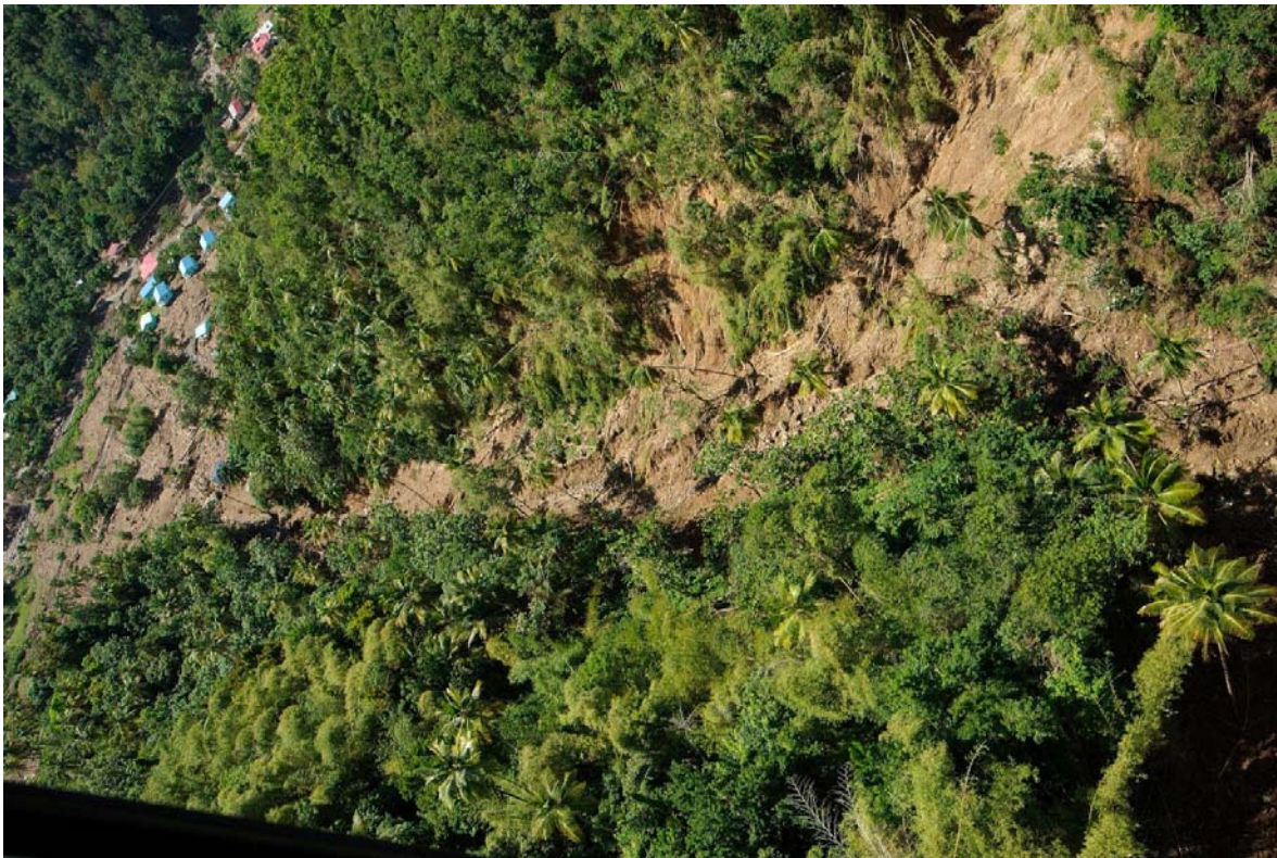
Top: Cresslands Development, looking toward Soufriere, Bottom: Looking down the path of flow slide toward the development
