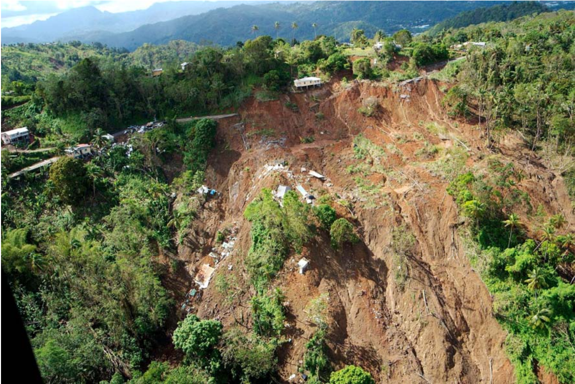
Guesneau: 150 m of Roadway in front of yellow house breached by landslide-I
