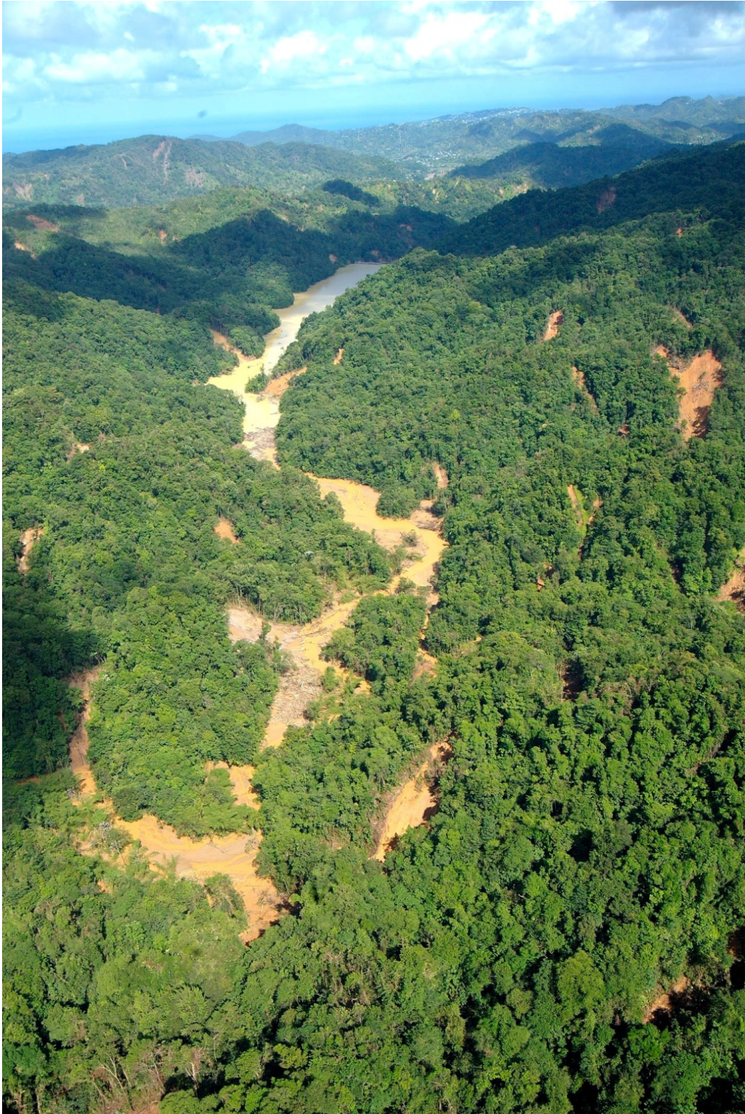
Roseau Dam, multiple debris flows in catchment area
