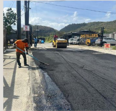
WEST COAST ROAD REHABILITATION- ROSEAU
