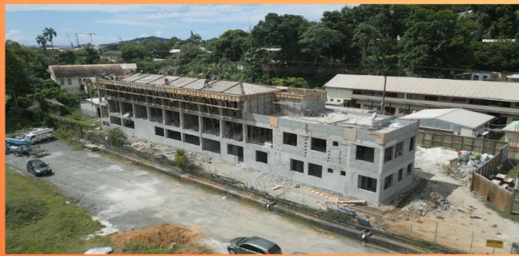
ENTREPOT SECONDARY SCHOOL - NEW WING
