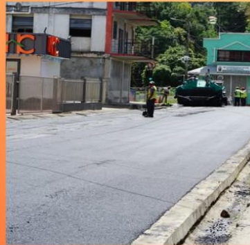
CHAUSSEE ROAD REHABILITATION
