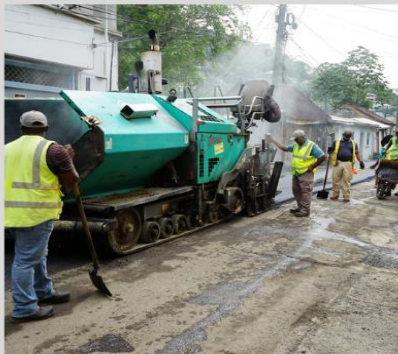
WATERWORKS ROAD REHABILITATION
