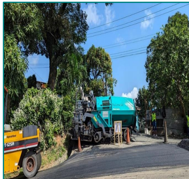
Road Rehabilitation Works - Bocage
