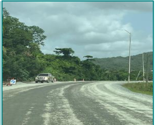
Millennium Highway - West Coast Road
