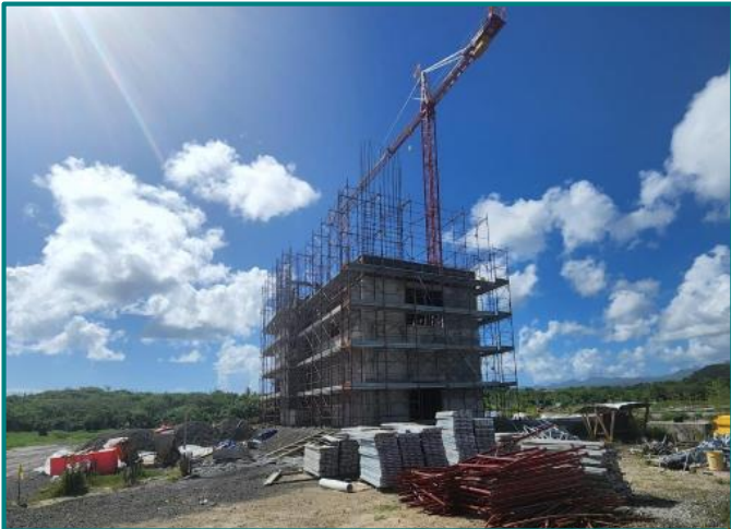
HIA Tower Construction
