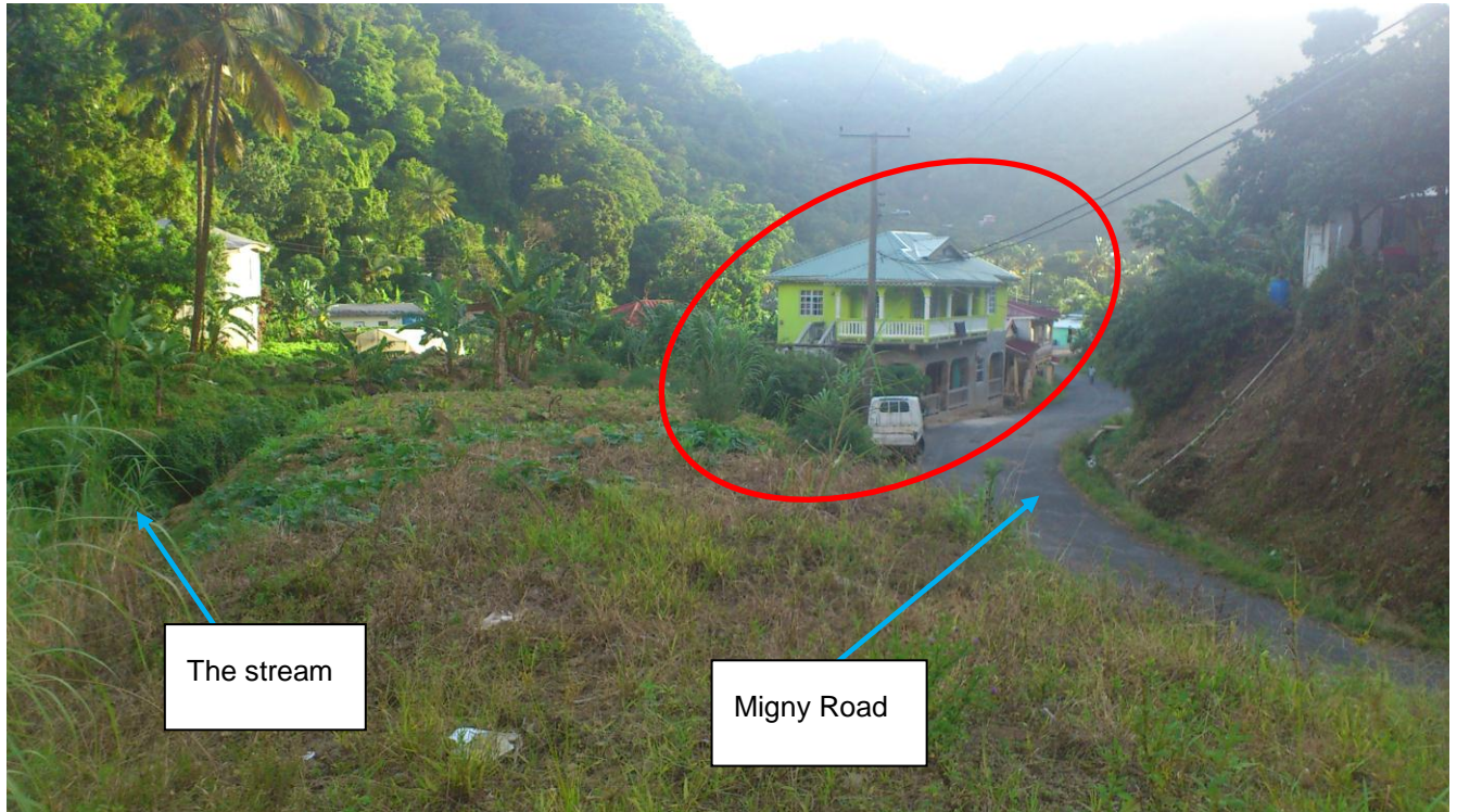
Figure 49 : Houses in Fond Saint Jacques to destroy -> all houses between the Migny road and the stream
