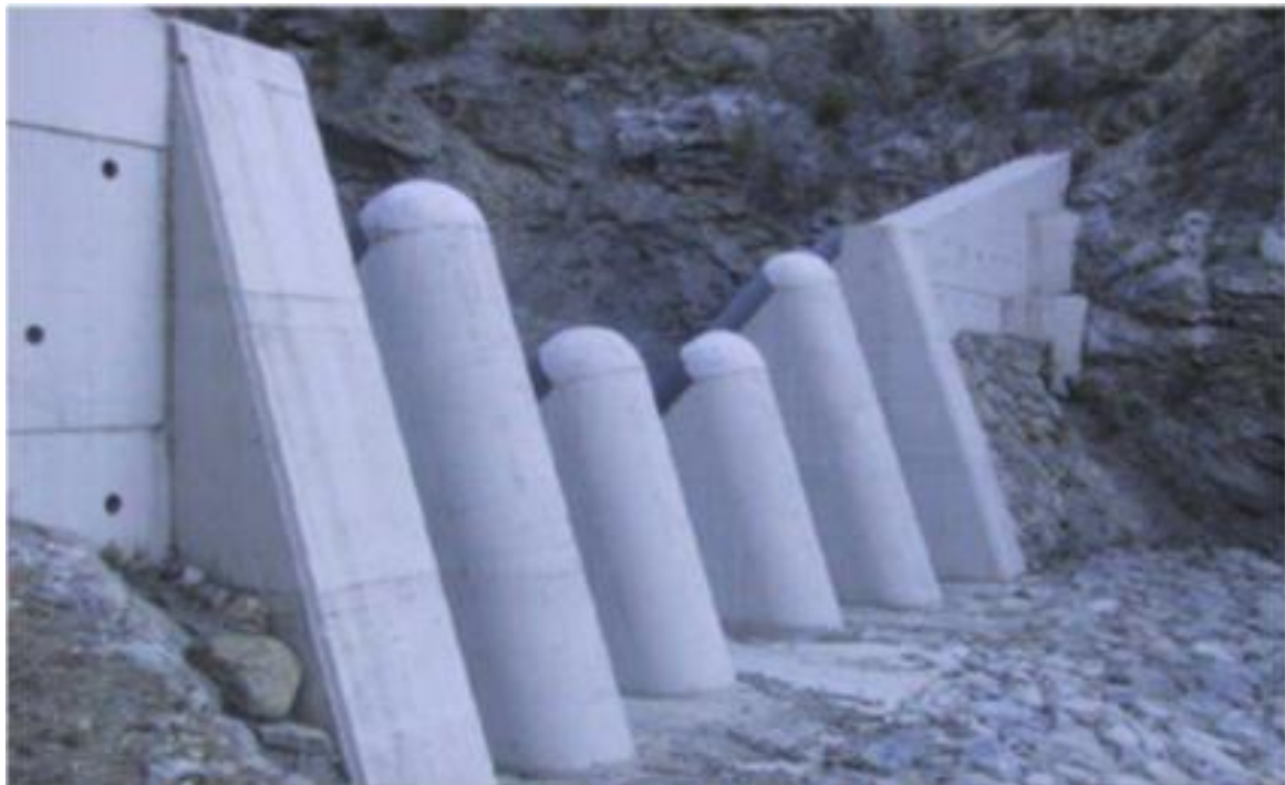
Figure 44 : view of a debris flow resisting jam trap
