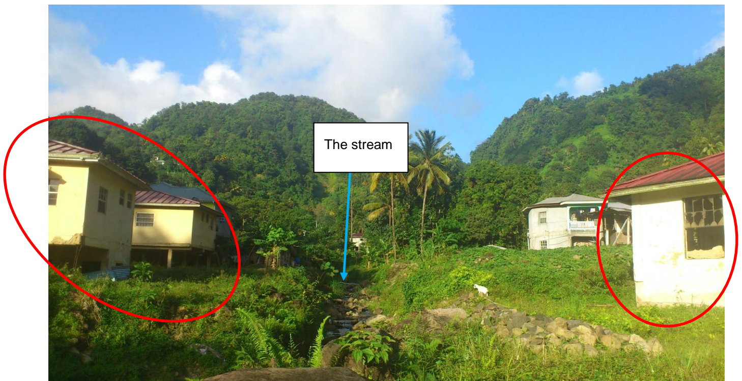
Figure 50 : Houses in Fond Saint Jacques to destroy view from the bridge 2b (see Figure 41 : Fond Saint Jacques critical infrastructures)
