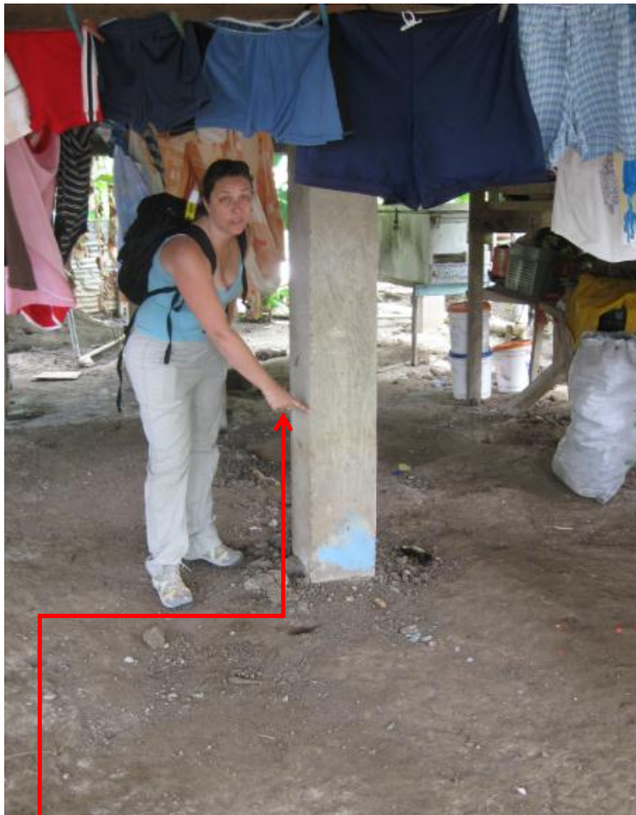
Measure the level shown on the pilar with the blue trace under the house left bank
