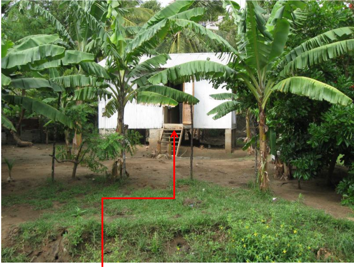
Measure the level of the last stair before the floor of the house right bank
