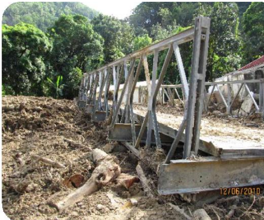
Figure 28 : photography of Fond Saint Jacques upstream bridge (road to Migny)
