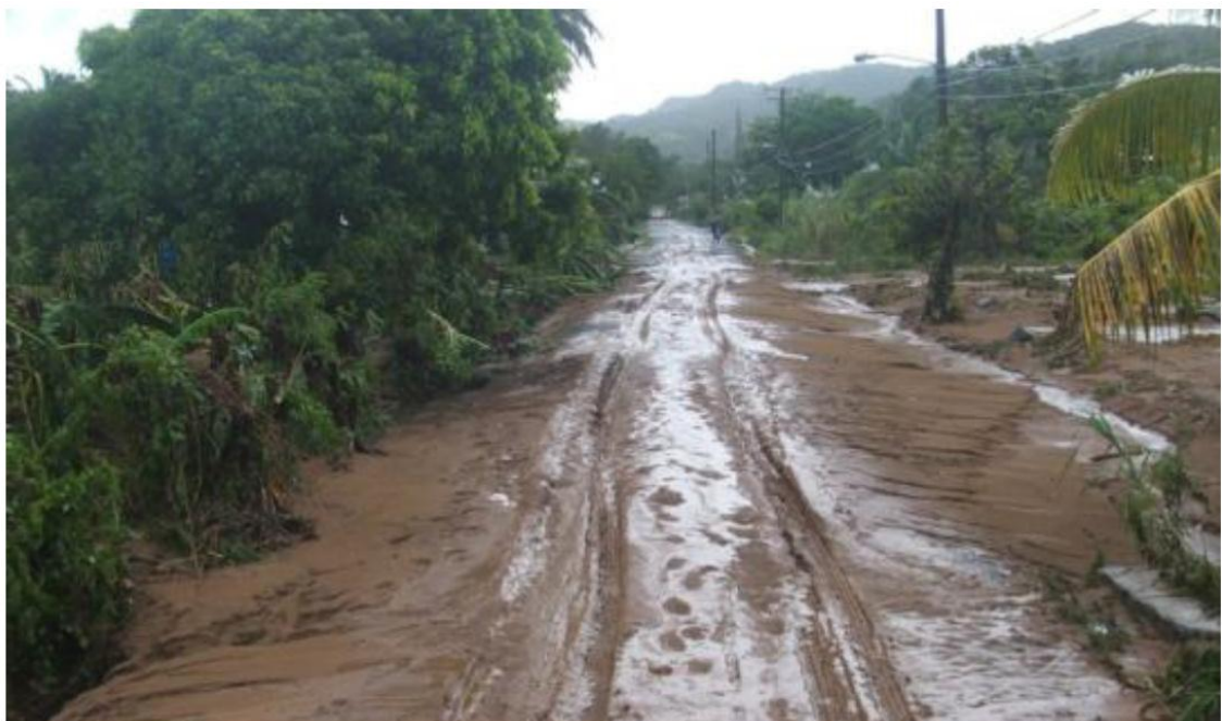
Figure 11 : Silt Deposit after Tomas in Mole Road
