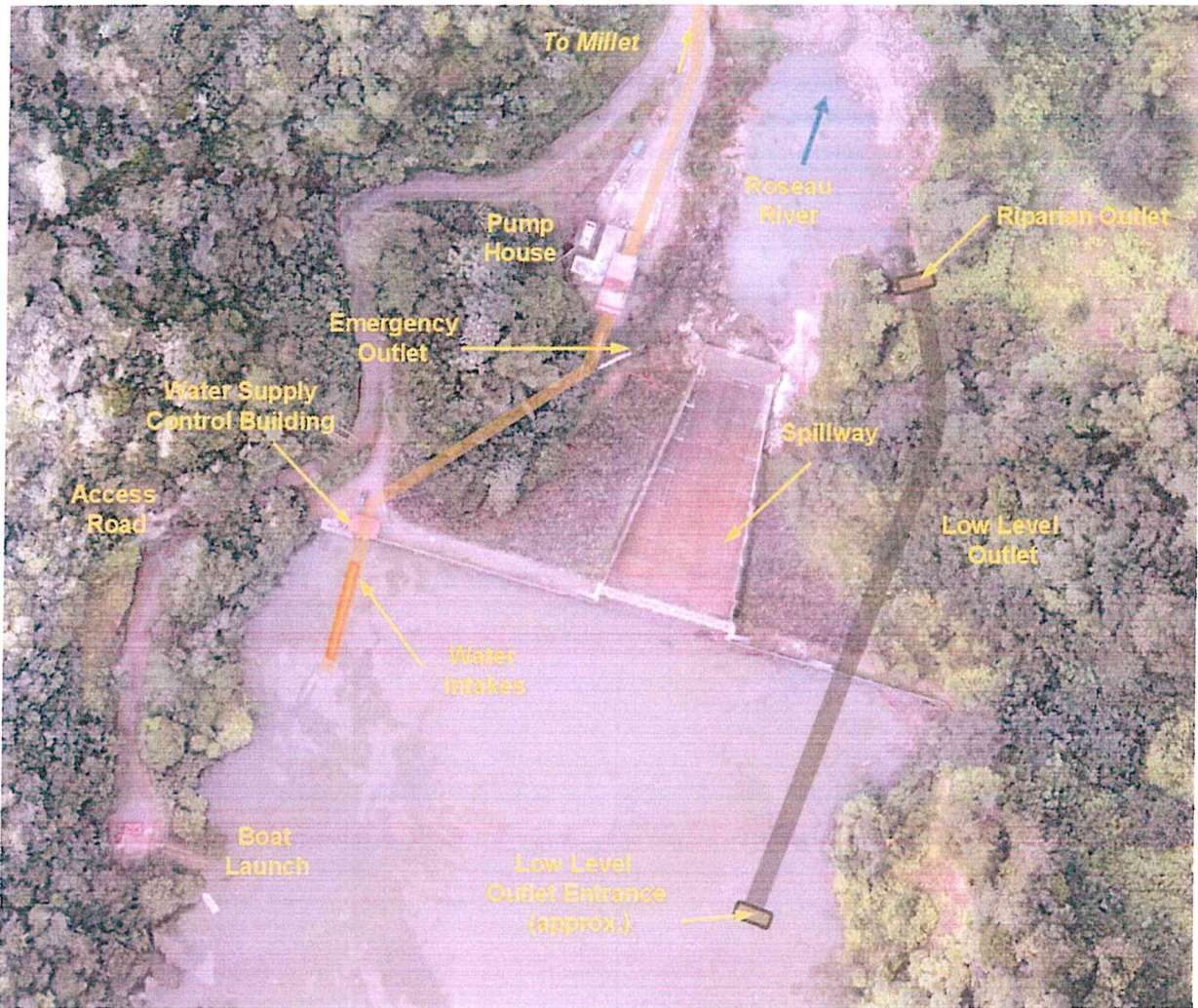
Figure 6: John Compton Dam General Arrangement (imagery from Golder UAV survey, October 2014)
