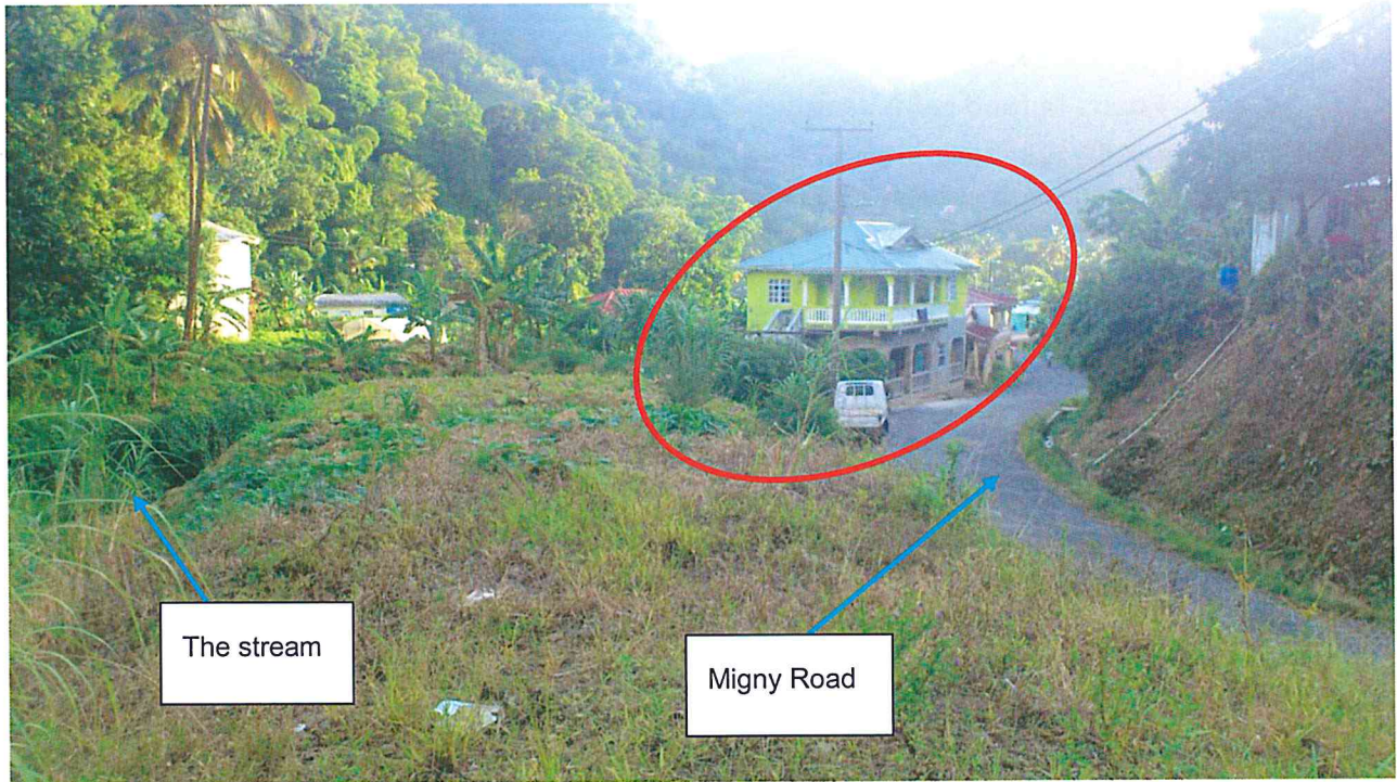
Figure 49 : Houses in Fond Saint Jacques to destroy -> all houses between the Migny road and the stream
