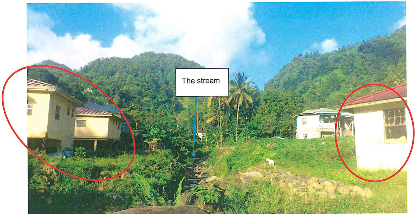
Figure 50 : Houses in Fond Saint Jacques to destroy view from the bridge 2b (see Figure 41 : Fond Saint Jacques critical infrastructures)
