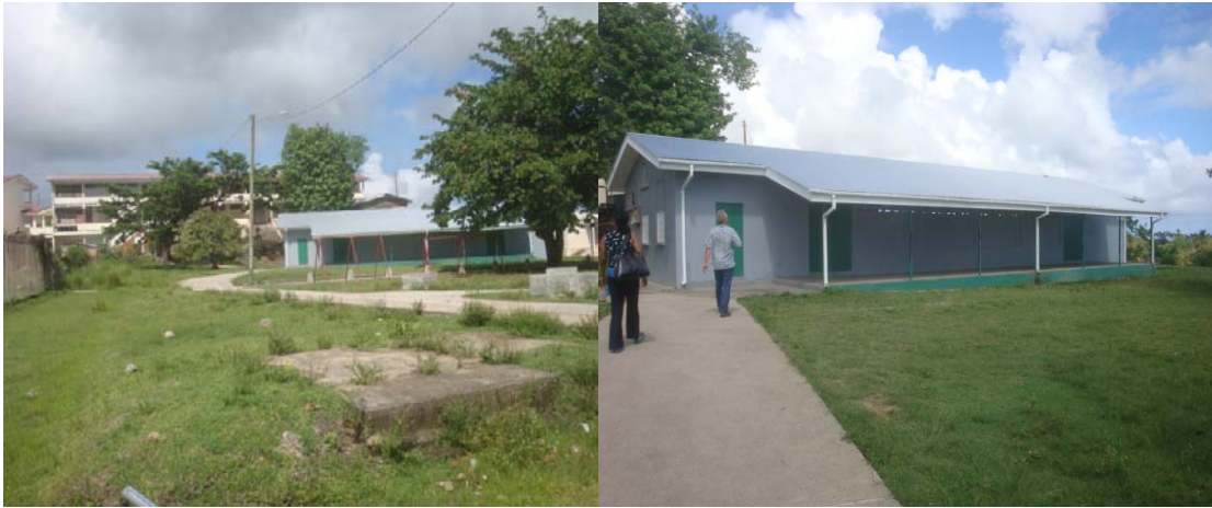
La Fargue Community Centre – conditions
