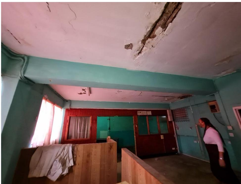
**Photo 20: Damage to soffit of concrete roof slab in 2 storey office section.**
