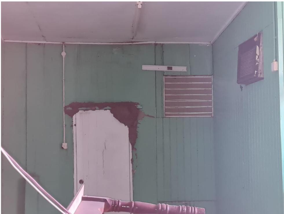
**Photo 18. Active termite nest above door in 2 storey office section.**
