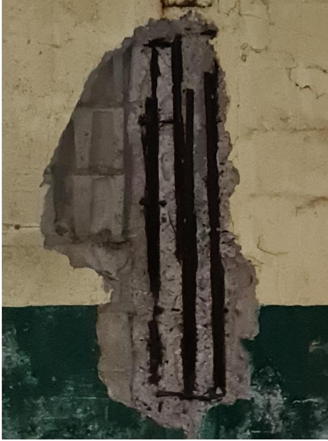
**Photo 13: Damage to stiffener column within blockwall.**
