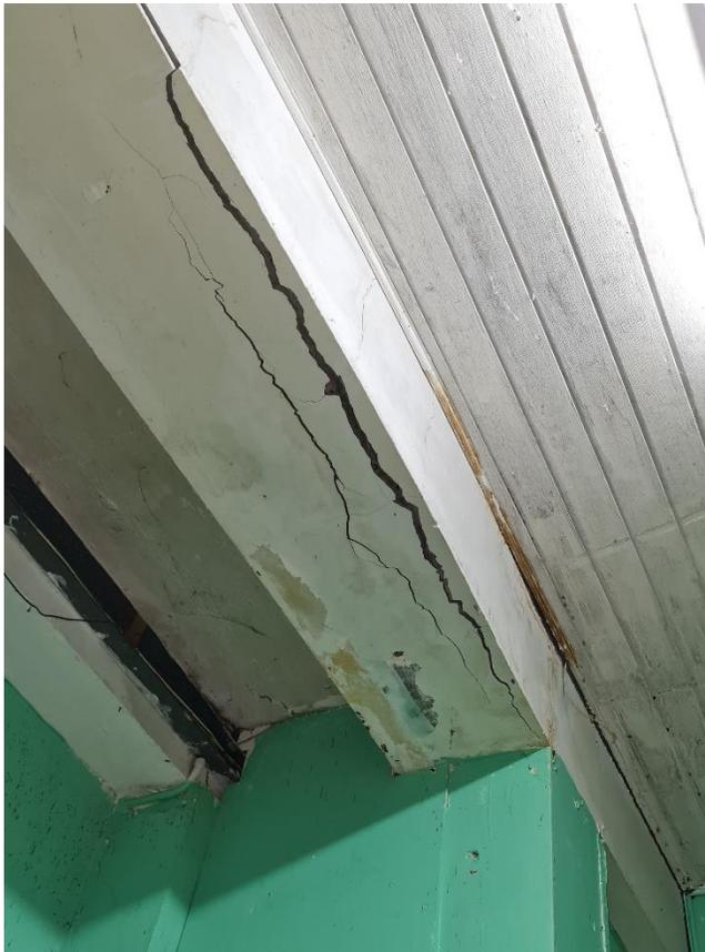
**Photo 9: Cracks in roof support beams.**
