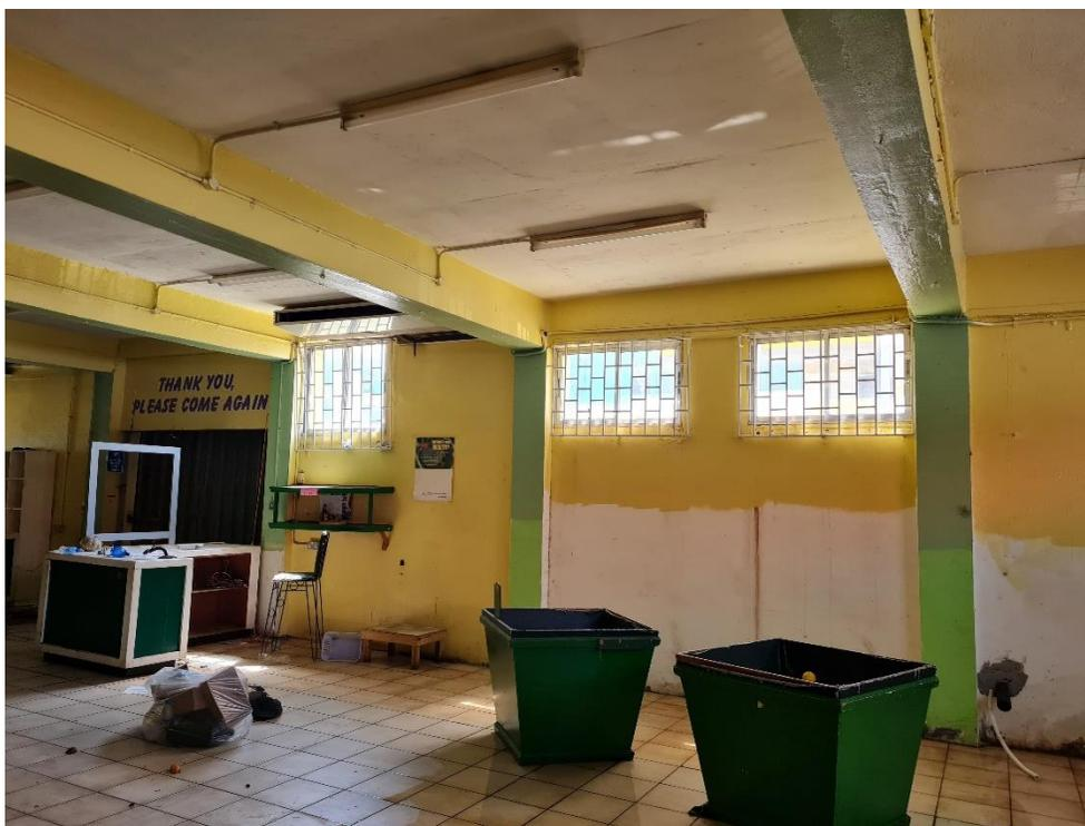
**Photo 4: Internal former shop space to the eastern side of the building. Note the exposed concrete slab soffits and beams.**
