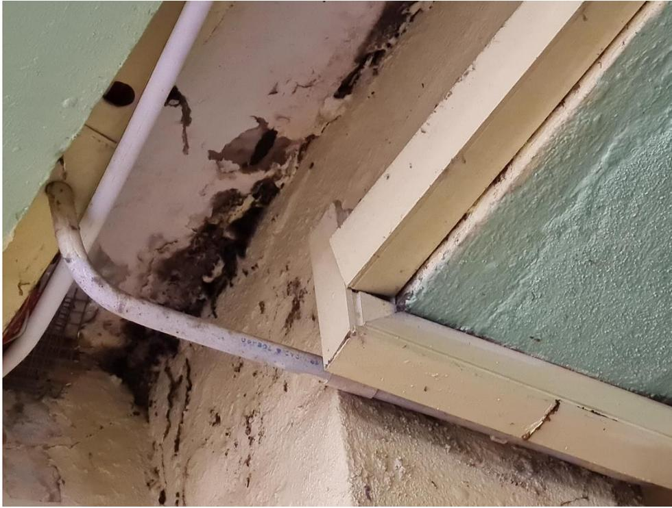
**Photo 7: Ingress of water from the roof slab above and presence of mold.**
