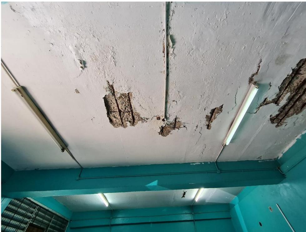
**Photo 8: Spalling of concrete from soffit of concrete roof slab.**
