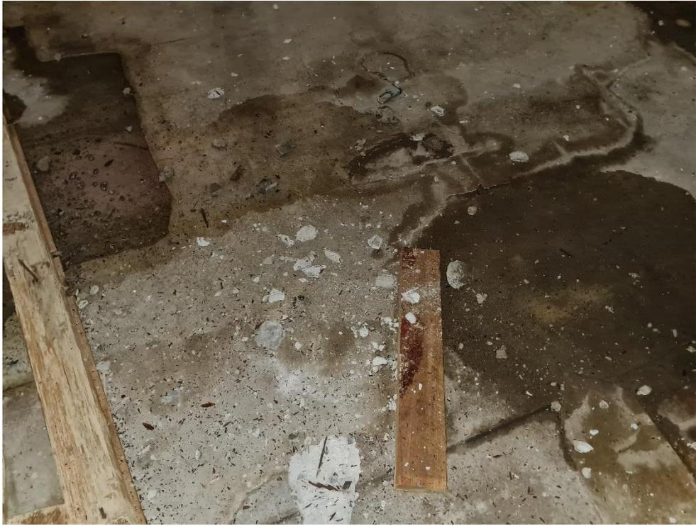
**Photo 17, Small chunks of spalled concrete on floor from ceiling above.**
