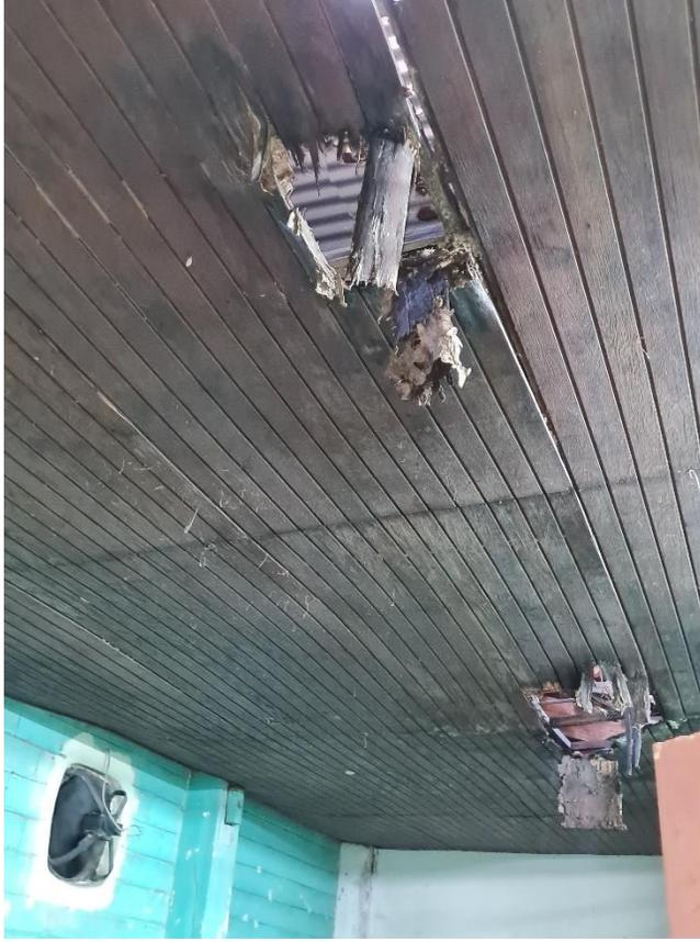
**Photo 11: Water damage to plywood ceiling.**
