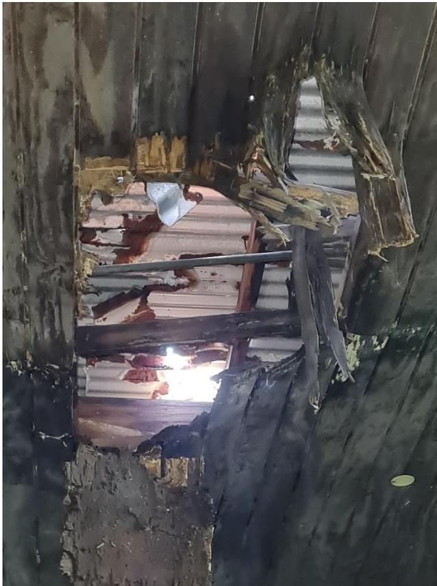
**Photo 12: Water damage to plywood ceiling and damage to roof sheathing.**
