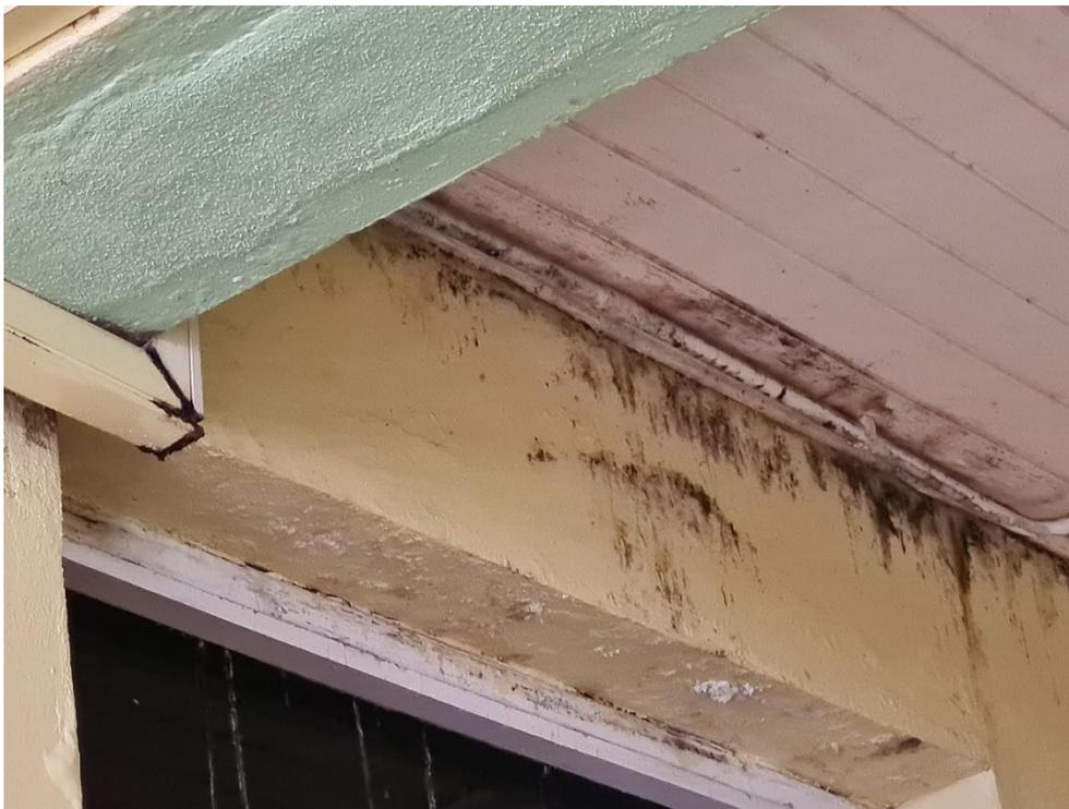
**Photo 6: Ingress of water from the roof slab above and presence of mold.**
