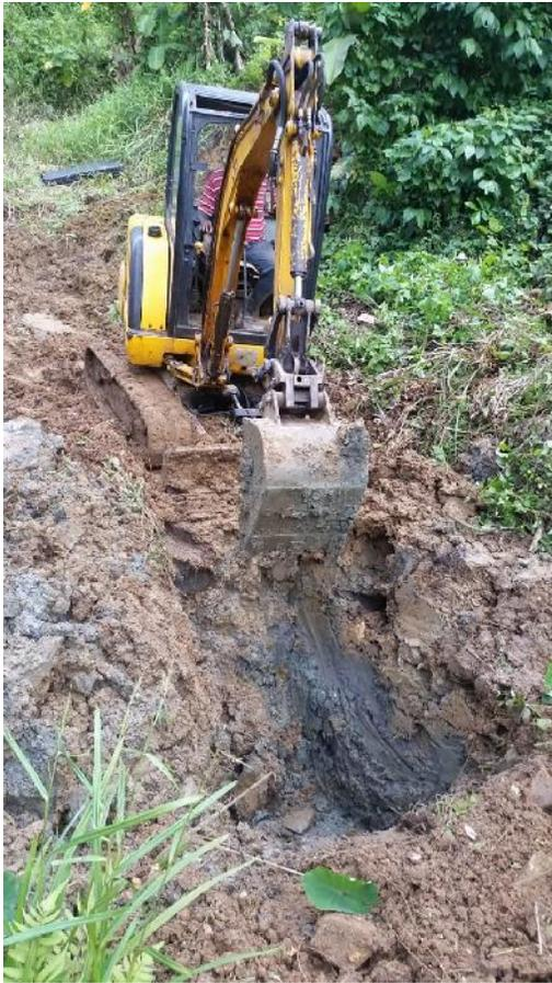
*Photo 1: Test Pit Excavation at T-Junction*
